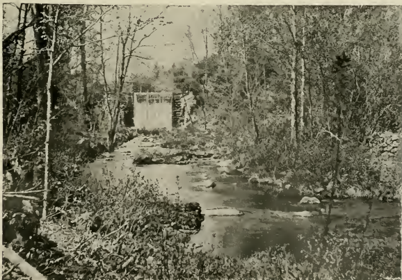
DAM AT UPPER RESERVOIR
